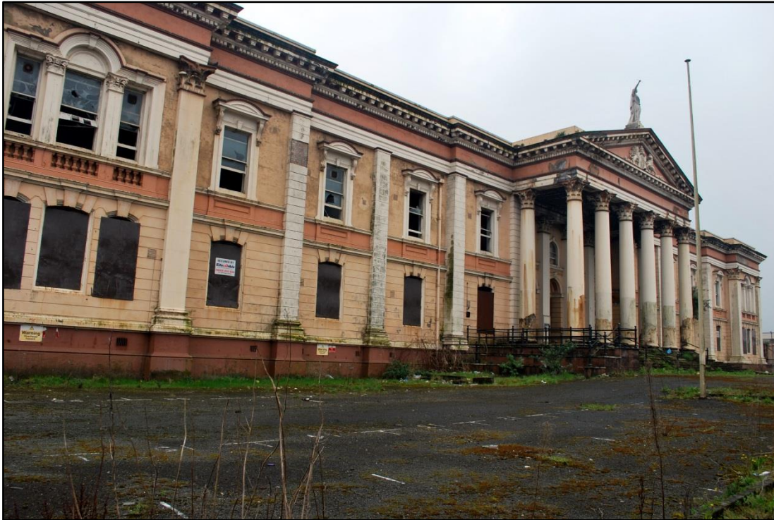
Fig. 36. Antrim courthouse, Crumlin Road, Belfast, from the east. Lanyon's original design was greatly altered and expanded in the early 1900s by Young & Mackenzie and has been abandoned since about the late 1990s. In recent years fires and vandalism have caused great damage to the interiors. Photograph by author, 2012.
