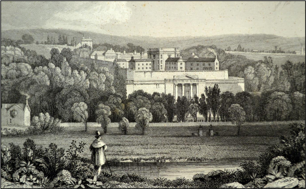
Fig. 45. Cork county gaol, from the city gaol, looking south, 1831. Behind the Greek portico, which survives, we can see Pain's radial cell blocks and the central-inspection hub. These were demolished around 1960. From G. N. Wright, Ireland illustrated from original drawings (London: Fisher, Son, and Jackson, 1831), pp. 66-67.
