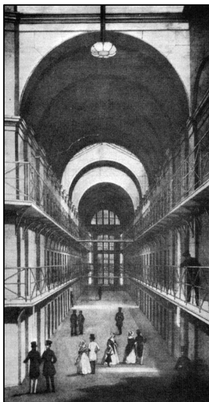
Fig. 10. Pentonville (the ‘model prison’), London, perspective view of interior. Joshua Jebb, 1840-2. On a much larger scale, Jebb demonstrated the logic and order of linking cells with the inspection hub via a large hall and a series of iron walkways (compare with Fig. 9). From Report of the surveyor-general of prisons on the construction, ventilation and details of Pentonville Prison, 1844 , H.C. 1844 (594), xxviii.
