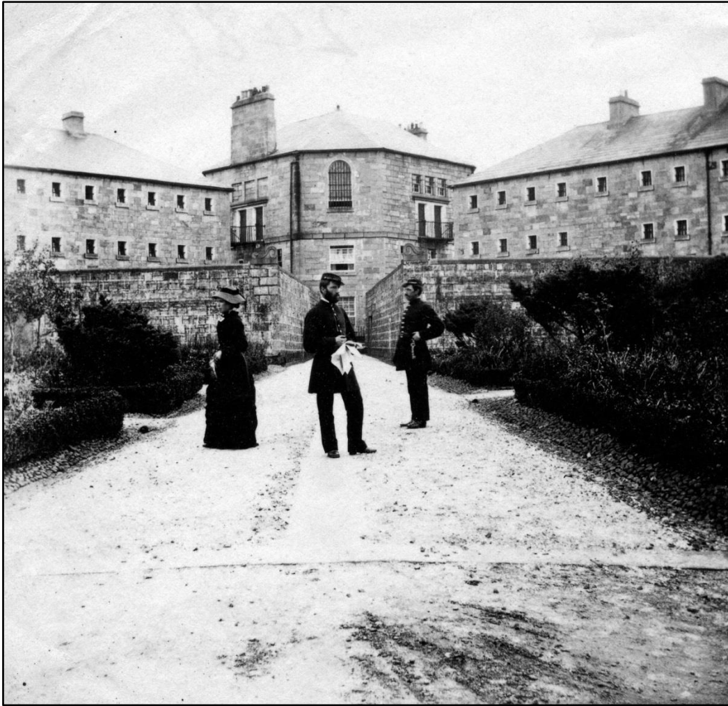
Fig. 47. Castlebar gaol, inspection building and two radial blocks, c. 1900 (by Thomas J. Wynne). The large radial-plan gaol marked a revolutionary change in the county's prison system and allowed proper classification and inspection for the first time. It was built with extensive government loans, which, it would appear, were never fully repaid. The three figures, a lady and two men, remain unidentified. Reproduced courtesy of Source Photographic Archives (Wynne collection).
