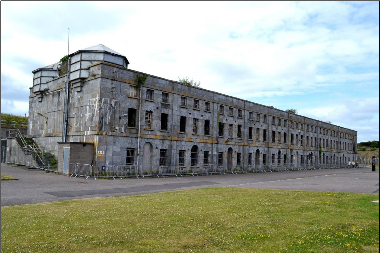
Fig. 32. Spike Island, Co. Cork, Fore Westmorland, part of barracks buildings, later used as a convict prison. Unlike Arbour Hill and Mountjoy, the prisoners on Spike Island were kept in buildings not initially designed for use as a prison. Many temporary prison buildings were erected on the site in the 1840s and 1850s. Photograph by author, 2017.
