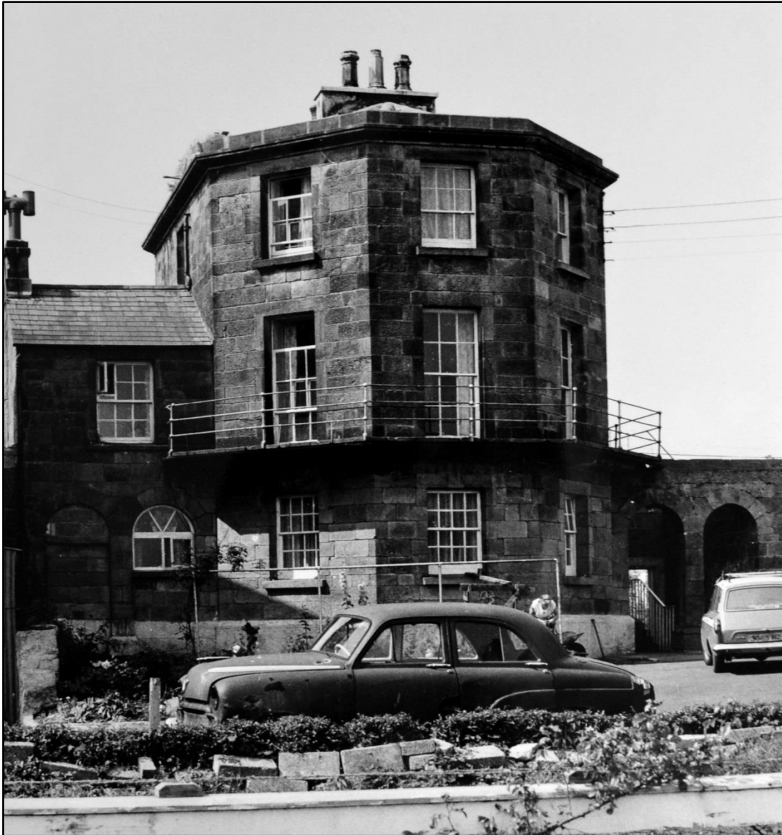
Fig. 12. The central inspection building, Omagh gaol, from the west, c. 1970. Now a domestic residence, this structure is the only surviving element of Hargrave's polygonal-plan additions to Omagh gaol in the 1820s. From its many windows, the gaoler could watch prisoners in the surrounding range of cells. Reproduced courtesy of the Irish Architectural Archive.
