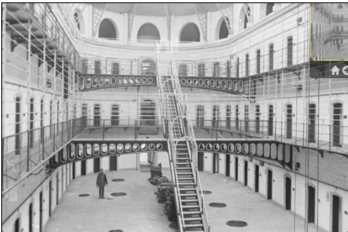
Fig. 47. Kilmainham gaol, separate-system block. McCurdy's celebrated rebuilding of Kilmainham gaol provided a distinctly Victorian image for an Irish prison, marked by its delicate iron brackets, arches, stairways, airy proportions, and roof lights. Reproduced courtesy of the National Library of Ireland.
