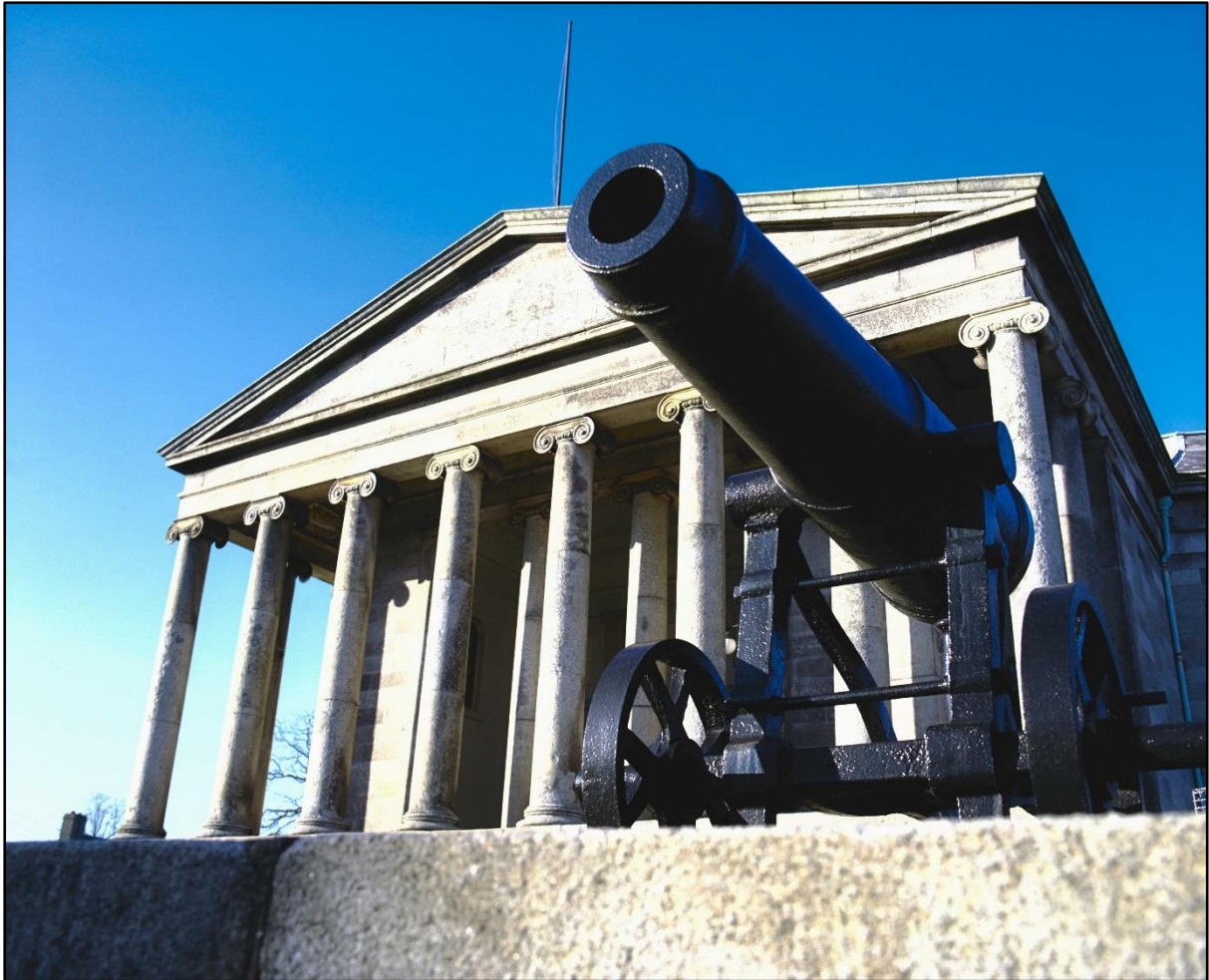
Fig. 27. Carlow courthouse, portico. The feverish building years of the early nineteenth century, fueled by wartime prosperity and later large government loans, culminated in the construction of Ireland's grandest and most sublime assize courthouse in one of its smallest counties. Photograph taken in 2007.
