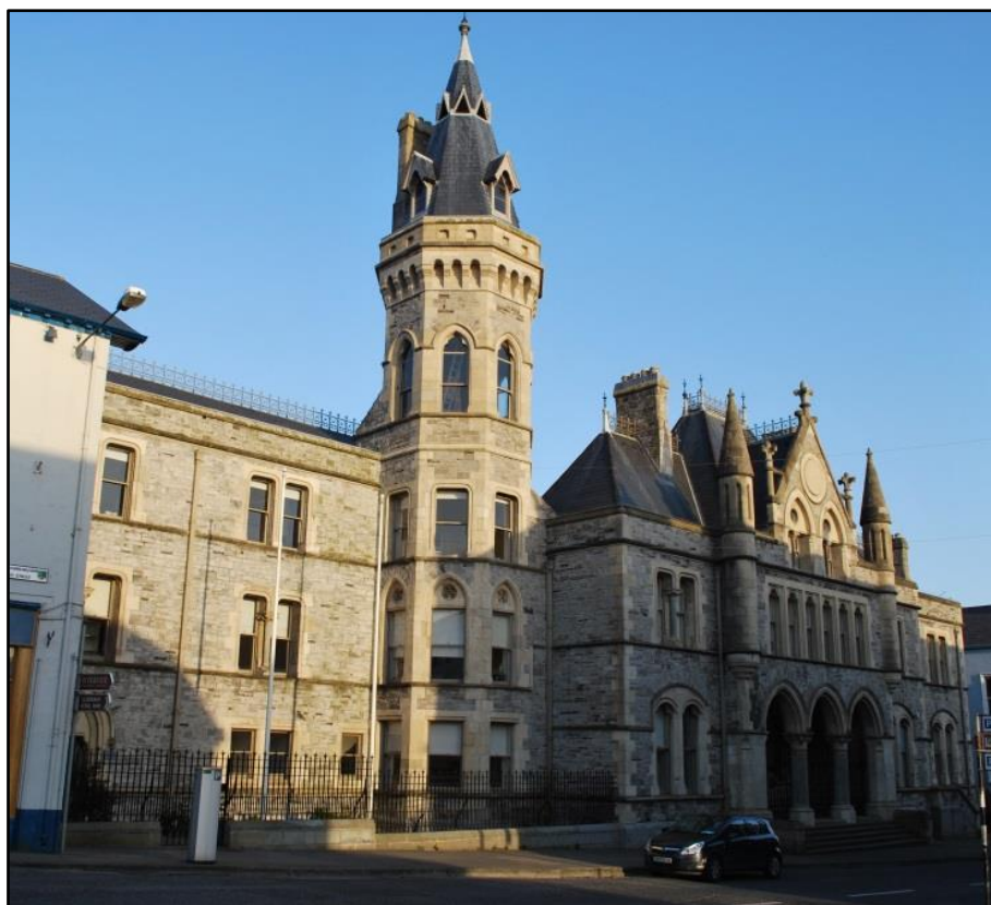
Fig. 37. Sligo courthouse, from the east. The grand jurors finally decided to replace their eighteenth-century courthouse in the 1870s with a Gothic Revival building on the same site designed by James Rawson Carroll. Photograph by author, 2012.
