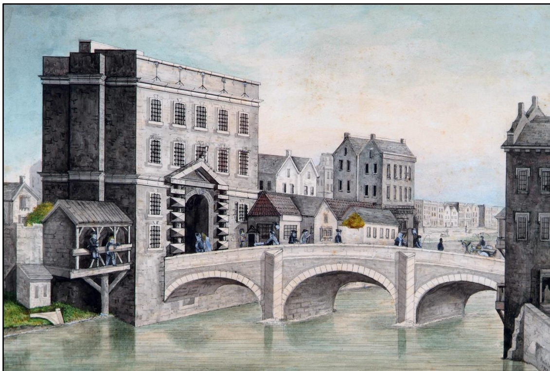
Fig. 4. John Fitzgerald (after Nathaniel Grogan), 'The South Gate and Bridge, Cork, 1797', c. 1850. Similar in scale and composition to the city gaol, this gatehouse held the county prisoners from the 1720s until the early nineteenth century. The rusticated columns and broken pediment of the passageway gave the gaol a false appearance of solidity, but prisoners found it rather easy to escape. Reproduced courtesy of the Crawford Art Gallery, Cork.
