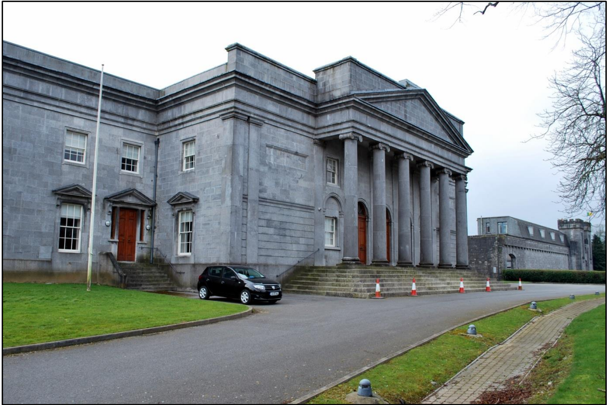
Fig. 4. Tullamore courthouse, by John B. Keane, with the Gothic former county gaol, by John Killaly, in the distance. Lord Tullamore feared that the opposing architectural styles would clash, and sketched a courthouse design more sympathetic to the gaol, but this was not built. The courthouse and gaol brought prosperity to the town and were the culmination of a fifty-year dispute between local elites. Photograph by author, 2013.
