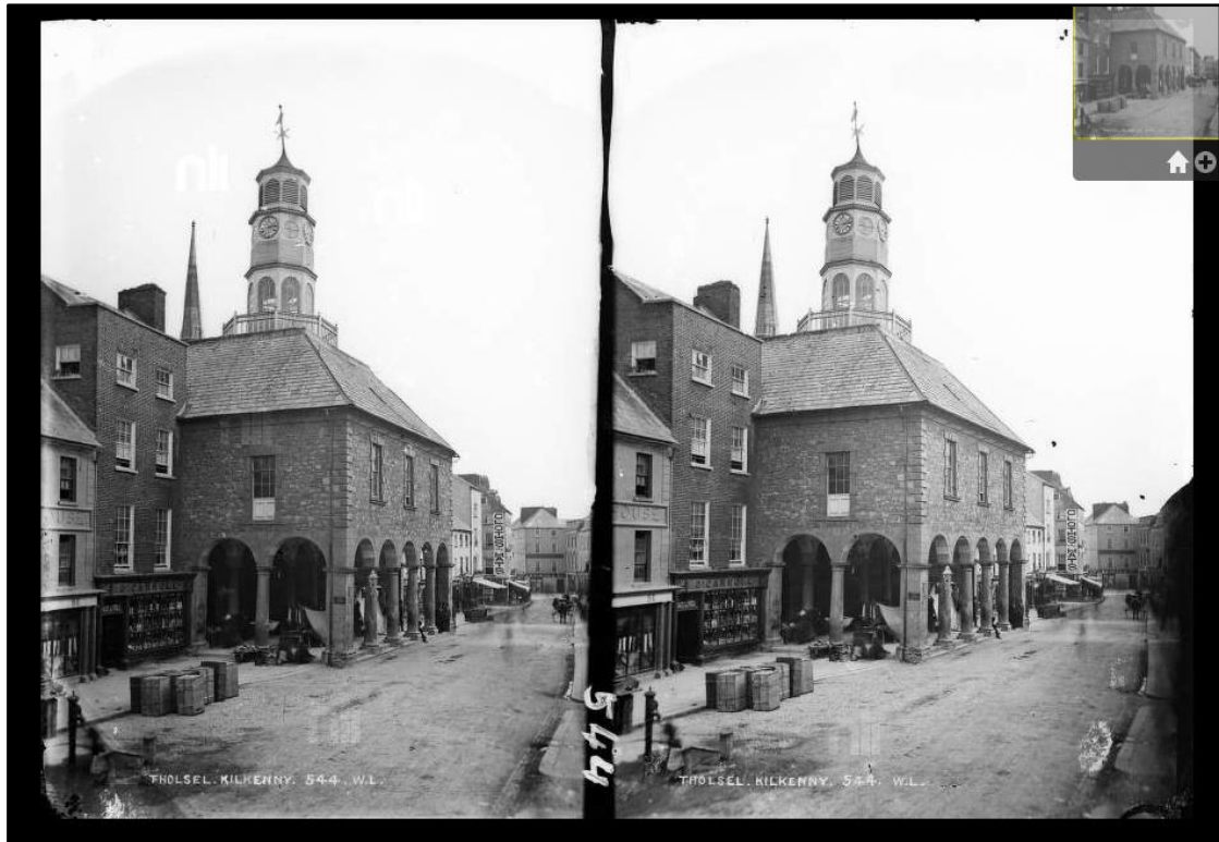
Fig. 7. Kilkenney's tholsel, c. 1900. A typical mixed-use markethouse and courthouse from the mid-eighteenth century. Traders were sheltered by the arcade, which so dramatically projects into the street, while court sittings were held upstairs. Reproduced courtesy of the National Library of Ireland.
