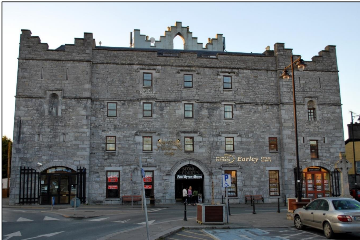
Fig. 20. Roscommon gaol, from the south. Built in the 1780s and 1790s, this gaol complemented the new courthouse built opposite it by the county grand jurors in the 1760s. Apart from its broad and rather theatrical façade, little was said in favour of the gaol’s design. Photograph by author, 2012.
