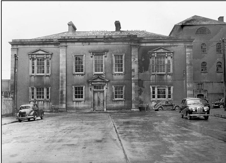
Fig. 28. Limerick city courthouse (left) and city gaol (right), as built, photograph c. 1950. These buildings were mostly demolished around 1990. The city courthouse was designed by James Pain in the 1840s in a simple and unornamented manner, unlike what Henry Hill had proposed a decade earlier. Reproduced courtesy of Sean Curtin and the 'Limerick: A Stroll Down Memory Lane' project.
