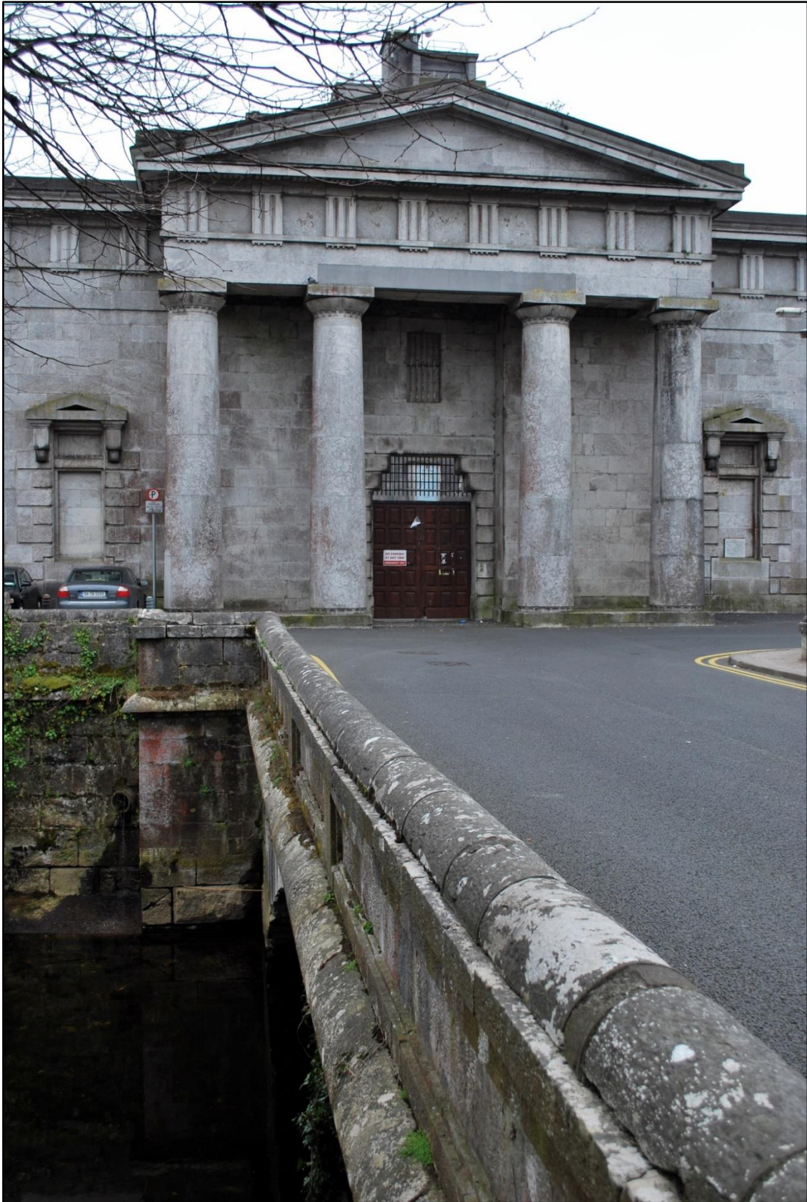
Fig. 46. Cork county gaol, portico, screen, and bridge over one channel of the River Lee. One of the most powerful essays in prison architecture in Ireland, Pain's portico adopted the Delian Doric order (likely via Stuart and Revett's The antiquities of Athens (1762)), while the corbelled arch over the main doorway was more Egyptian in inspiration. Contemporary observers as well as later critics have admired the composition. Photograph by author, 2013.
