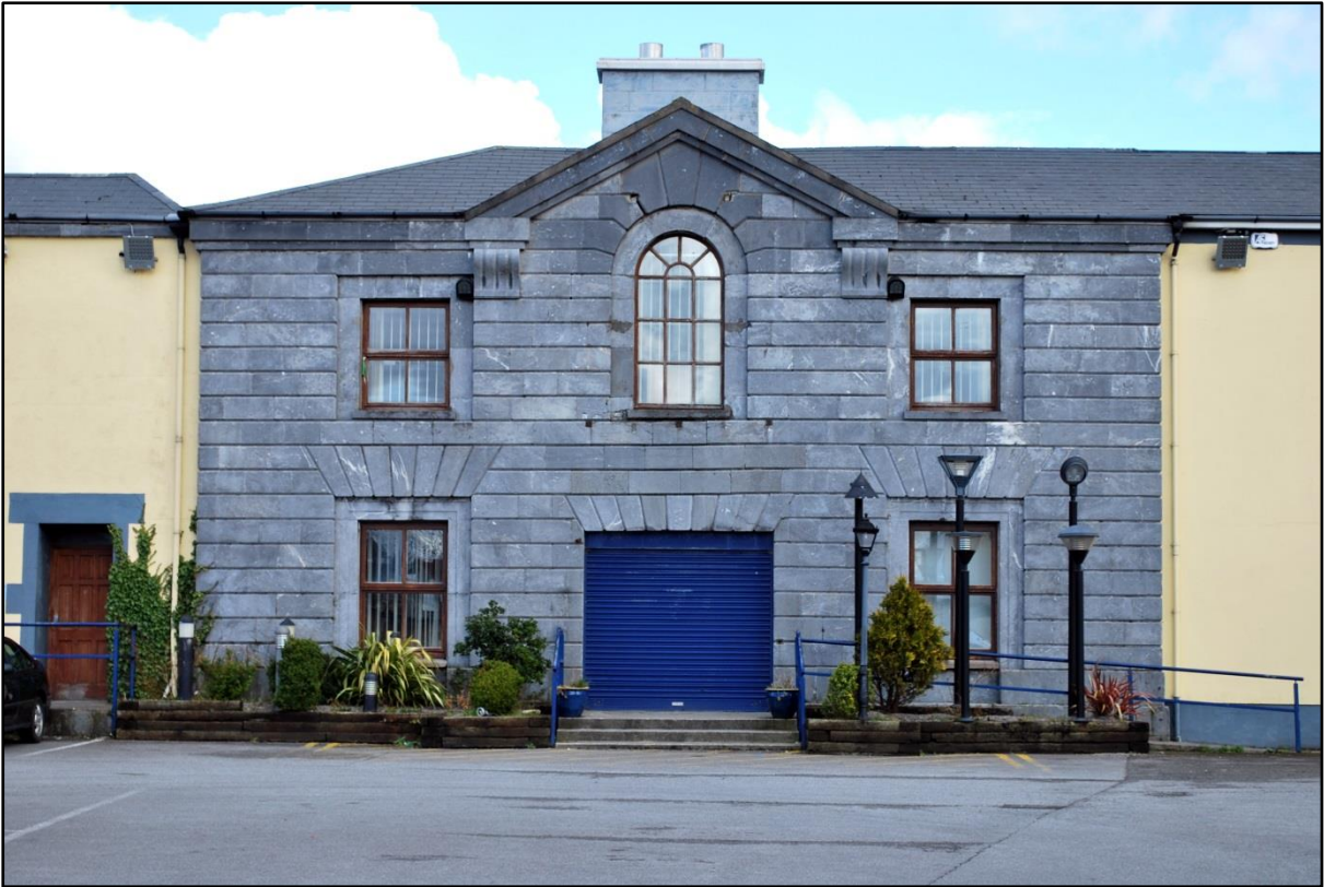
Fig. 24. Tralee gaol, entrance gateway, from the west. Today only this block and part of the boundary wall survive. Morrison's use of rustication was plainer and less intimidating than that in many other gaols built at the same time. Photograph by author, 2013.
