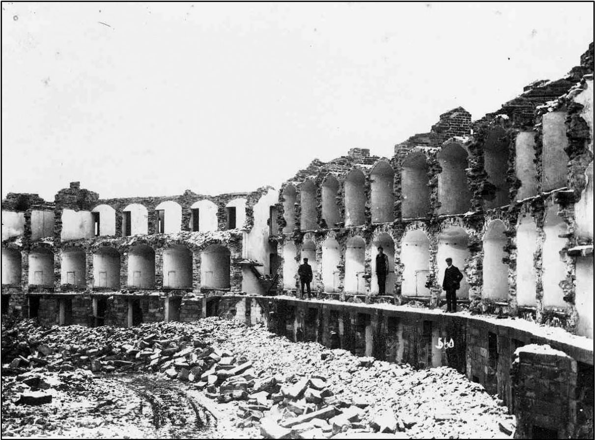
Fig. 14. Lifford gaol, Co. Donegal, under demolition, c. 1907. This rare photograph shows the stone and brick construction of Hargrave's walls and floors. These made the new gaols of the 1820s more secure and fire-proof than earlier buildings. These men had much hard work ahead of them. Reproduced courtesy of Donegal County Archives.
