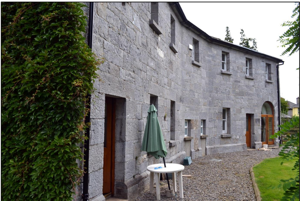
Fig. 21. Athy gaol, from the north-west. Hargrave's small, two-storey gaol was well built using local limestone. Today only a small portion of the cell block remains intact. Photograph by author, 2014. Reproduced with the permission of the present owners.
