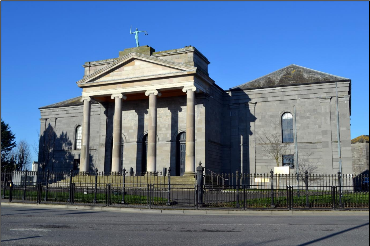
Fig. 18. Nenagh courthouse, from the south-east. Keane mixed local limestones and sandstones in the design of the main façade. The portico was substantially rebuilt in the 1890s, and the central sculpture of Justice is a much more recent and rather underwhelming addition. Photograph by author, 2017.
