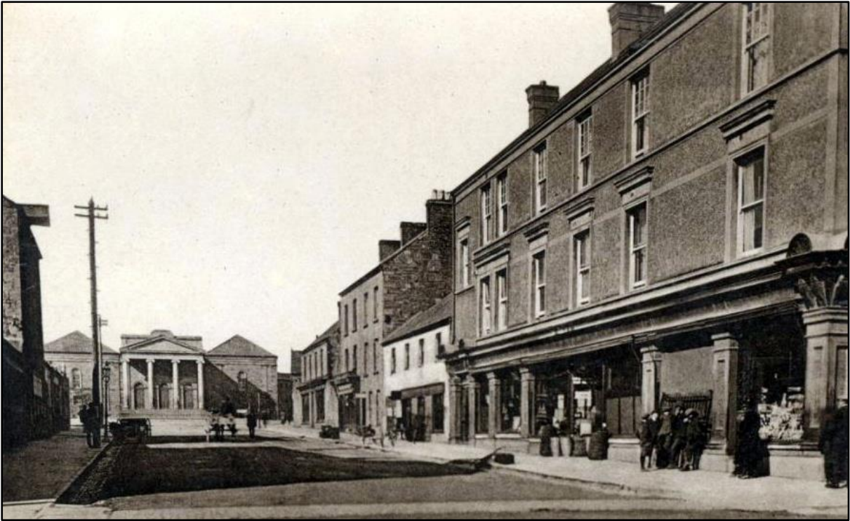
Fig. 16. Nenagh courthouse and Peter Street, c. 1900. John B. Keane gave his building an advantageous site on a newly planned street, terminating it axially with its tetrastyle portico. Reproduced courtesy of Tipperary Studies, Tipperary County Council Library Service.
