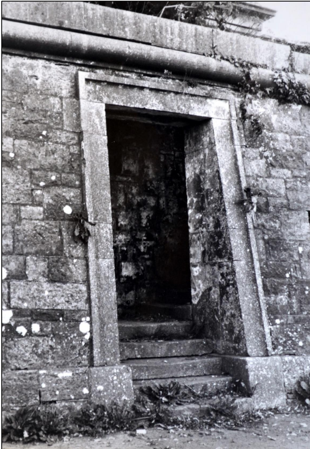
Fig. 31. The entrance steps and terrace wall, Trim gaol, from the north-east, 1981. Carved into the earth, the double staircase was entered through a doorway with inclined jambs and gave access to the elevated main entrance to the gaol behind (visible in the top right). Reproduced courtesy of the Irish Architectural Archive (photograph by Geoff White).
