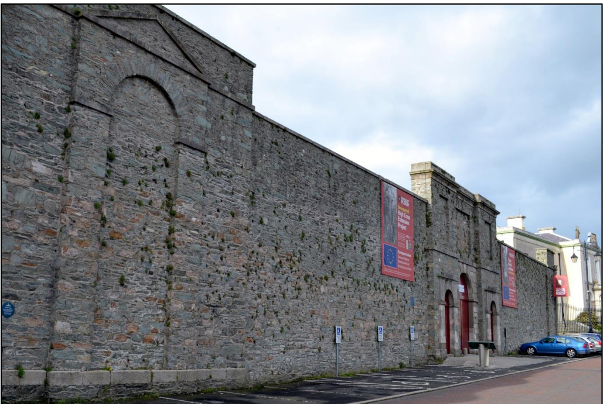
Fig. 18. Downpatrick gaol, from the south-west. Built by Charles Lilly between 1789 and 1796, the new gaol for County Down was similar to Kilmainham in many aspects of its plan; both derived from the principles established by Howard in the previous decade. The gaol survives today as a museum, with the assize courthouse visible in the distance. Photograph by author, 2014.
