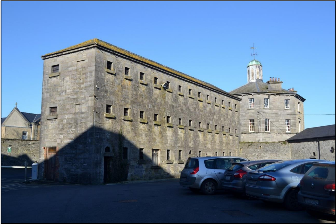
Fig. 28. Nenagh gaol, a surviving cell block, from the south. The narrowness of this block indicates its asymmetrical corridor-and-cell layout, while the alternating window-sill heights on the ground floor reveal the original intended function of the ground floor rooms as day-rooms rather than separate-system cells (compare with Figs. 8, 13). When complete in 1843, this design was seen as old-fashioned and inconvenient. Photograph by author, 2017.
