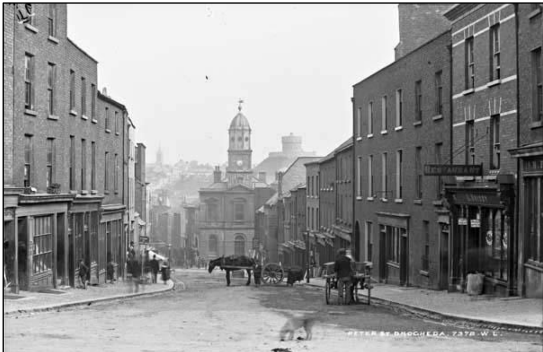
Fig. 8. Drogheda's tholsel, c. 1900. The grand jury of the town of Drogheda held jurisdiction over one of the smallest administrative counties in Ireland. Their combined markethouse and courthouse was located at the crossing of the town's principal streets. Reproduced courtesy of the National Library of Ireland.
