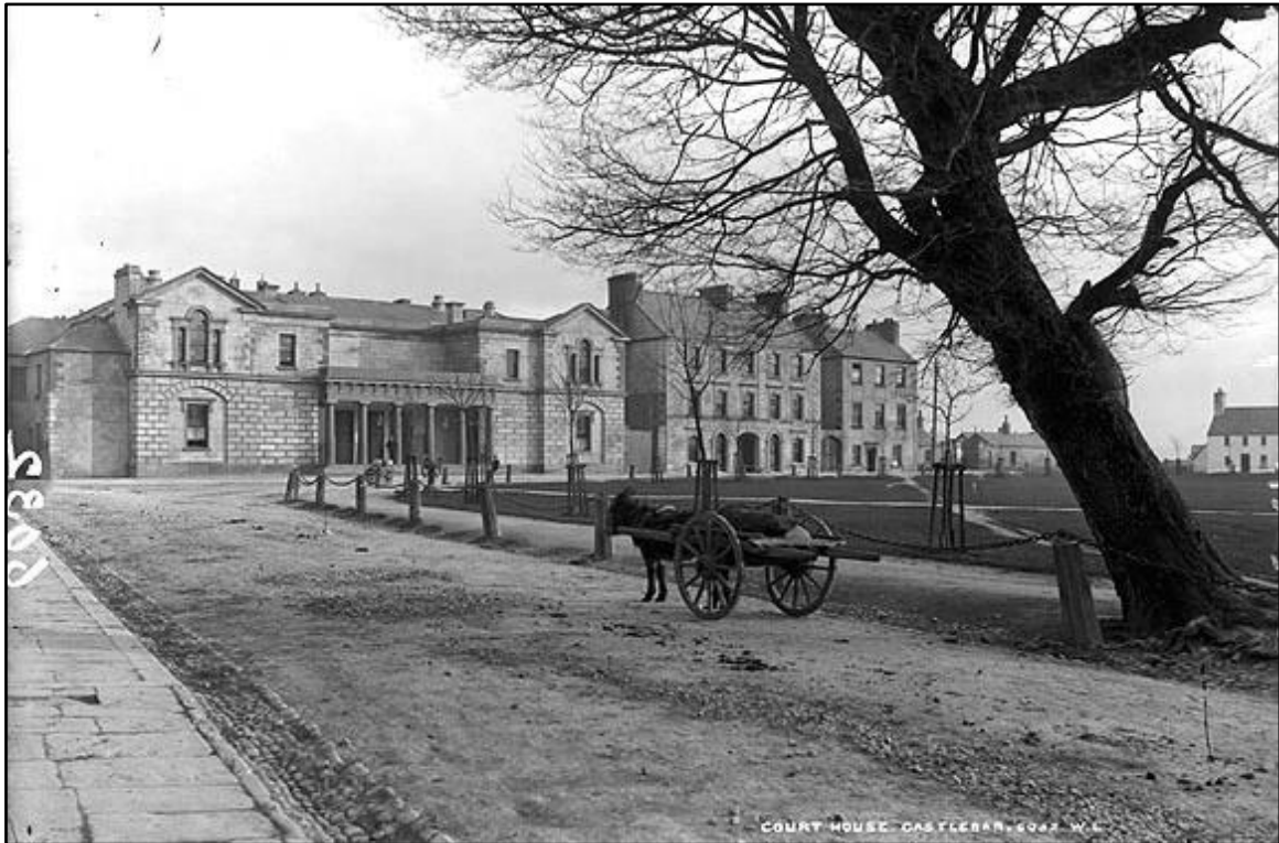
Fig. 14. Castlebar courthouse, c. 1900. Built by George Papworth in the early 1820s, it was extensively altered in the late 1850s. The central Doric portico was one of the first in Ireland to have been built of cast iron. When it was complete, there were clustered around this little green: two army barracks, two hospitals, the county gaol, and a Protestant church – all the perquisites of a county town. Reproduced courtesy of the National Library of Ireland.
