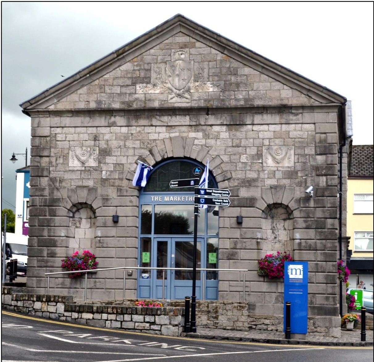
Fig. 20. Monaghan markethouse (1792), with the pediment displaying the coat-of-arms of the Westenra family, the proprietors of the town and one of the more influential political families in the county. Photograph by author, 2014.
