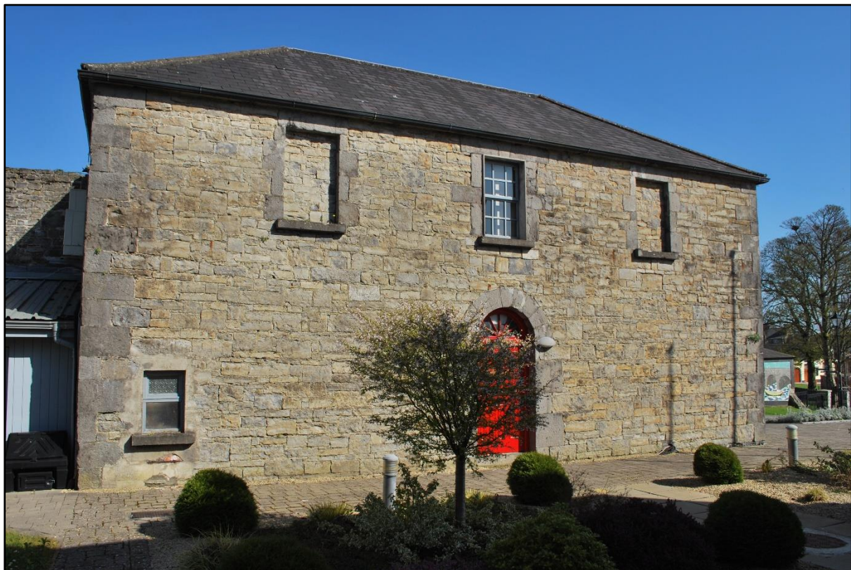
Fig. 10. Carrick-on-Shannon gaol, Co. Leitrim. A small remaining part of the former county gaol, located adjacent to the assize courthouse. Photograph by author, 2012.
