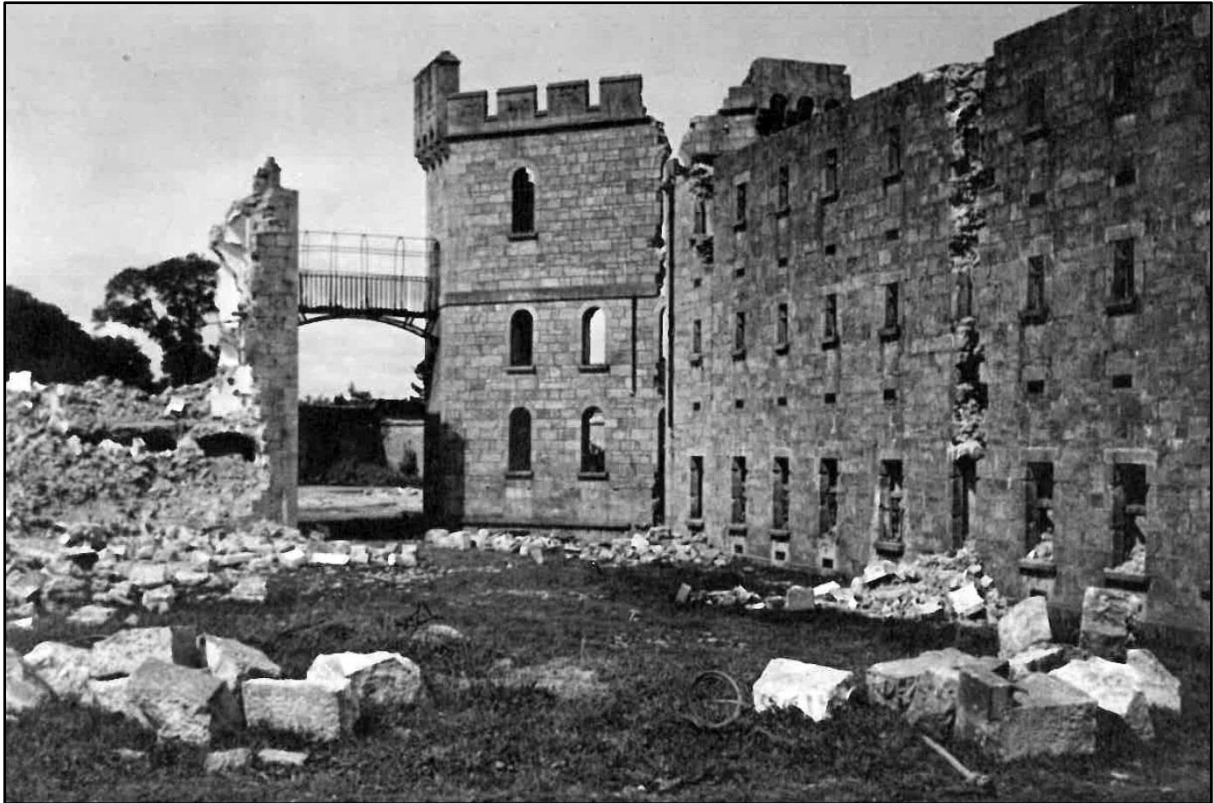
Fig. 38. Tullamore gaol, c. 1930s. The half-ruined central inspection building, in a Gothic style matching the façade, was connected to the radial cell blocks by iron bridges, of which one is visible here. The gaol was demolished some years after it was damaged during the War of Independence and Civil War.
