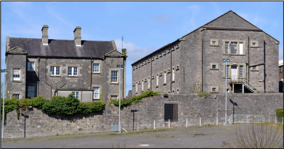
Fig. 13. Enniskillen gaol, separate-system block and infirmary, from the east. Today, the older parts of the gaol have been demolished but Farrell's additions from the 1840s remain remarkably intact. The large central hall of the cell block to the right is apparent from the arrangement of windows at the gable wall, while the smaller windows of the cells run down either side of the façade. Photograph by author, 2014.
