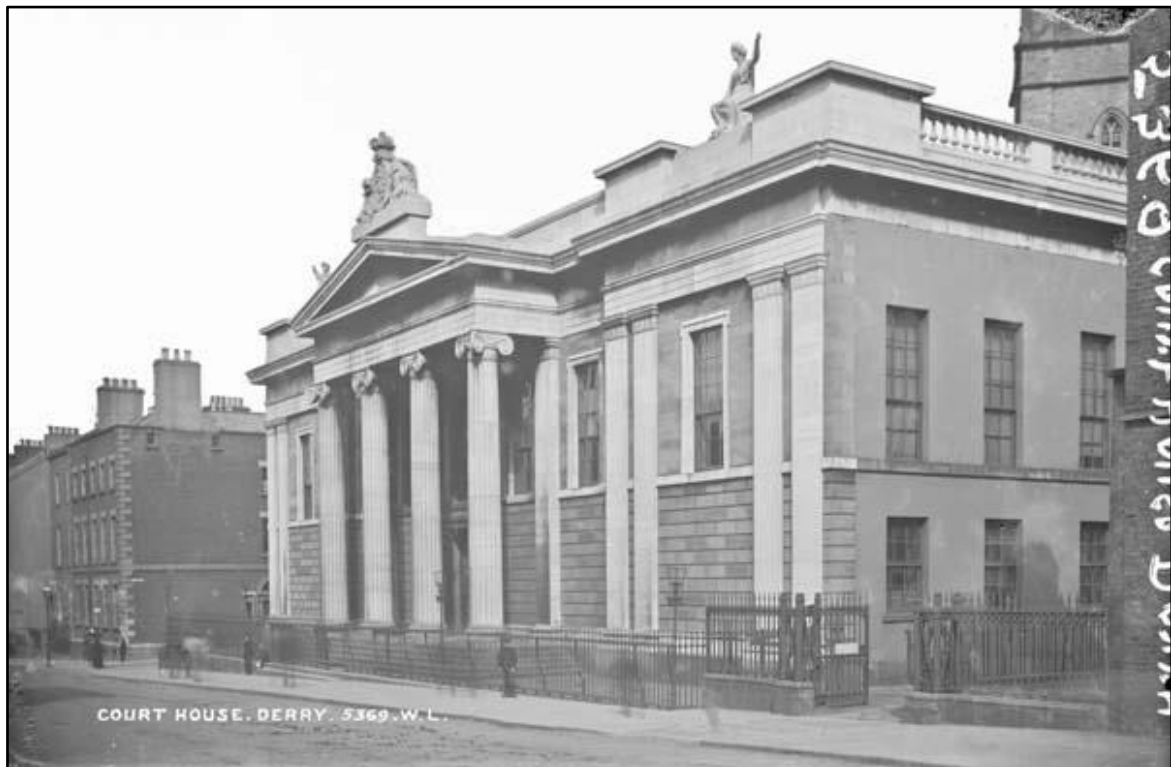
Fig. 45. Derry courthouse, c. 1900 (and largely as it appears today). Despite the grandeur of the building, the grand jury's choice of site was inferior to those of many neighbouring counties at this time. In the background the tower of the cathedral. Reproduced courtesy of the National Library of Ireland.
