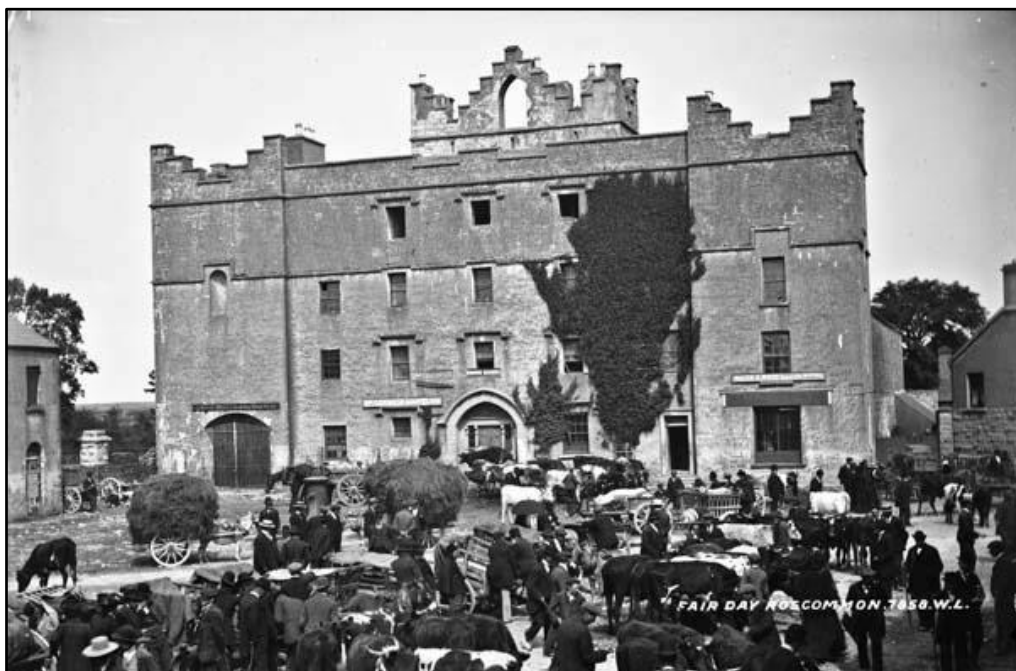
Fig. 15. Roscommon gaol and marketplace, c. 1900. Ensor's courthouse looked out onto the county gaol and a cattle market as in this late nineteenth-century view. In the 1820s both courthouse and gaol were relocated elsewhere in the town (see Chapter 2). Reproduced courtesy of the National Library of Ireland.
