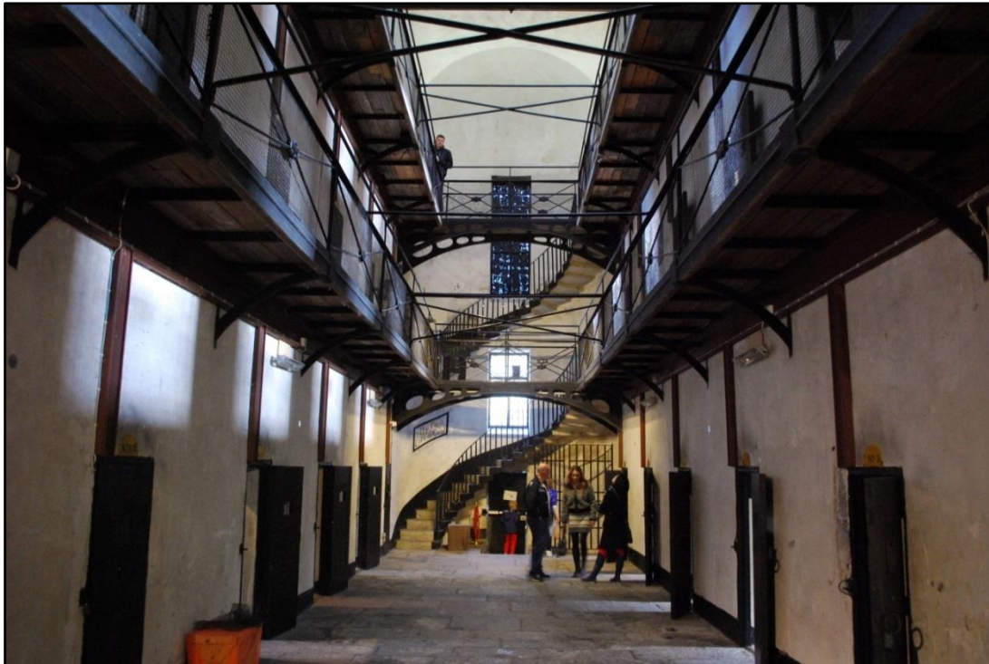
Fig. 9. Wicklow gaol, separate-system cell block, by John Semple, from the west. Instead of a narrow series of corridors that led to single rows of cells, as in earlier radial-plan prisons, Wicklow's cell block was designed with an airy, top-lit hall and iron mezzanine walkways that gave access to large cells on both sides. Following Pentonville, this layout allowed new levels of separation and inspection of prisoners (compare with Fig. 10 below). Photograph by author, 2013.
