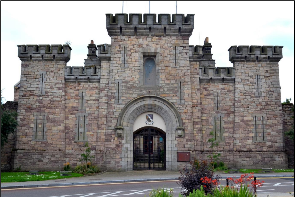
Fig. 16. Wexford gaol, from the north. Designed by John Semple and built between 1843 and 1846, this extravagant two-dimensional Gothick gateway led to a much plainer separate-system cell block behind that was similar to those built in Wicklow and Enniskillen at this time. Photograph by author, 2014.
