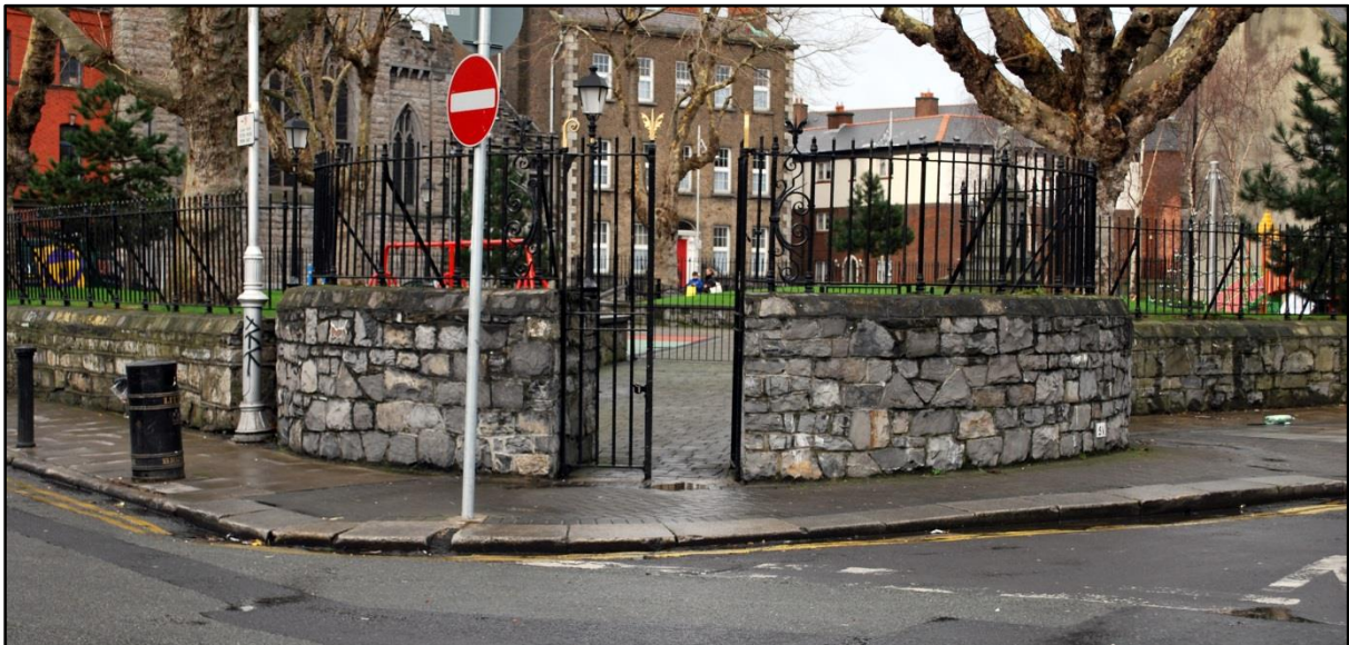
Fig. 35. St. Michan’s park, Green St., Dublin, from the south-east. Dublin’s Newgate gaol stood on this site between 1773 and 1893; today only the base of one of the corner turrets remains (though heavily rebuilt; compare with Chapter 4, Figs. 7-9). Photograph by author, 2014.
