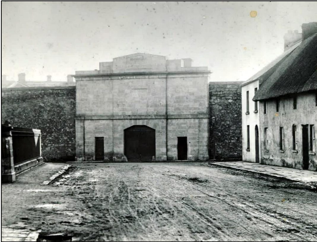
Fig. 18. The entrance gateway, Mullingar gaol, from the south, c. 1900. In the 1830s, the old and new parts of the gaol were brought together, and an entrance gateway rebuilt. This austere façade, since demolished, had a simple inscription in its pediment, 'MDCCCXXXVI'. Reproduced courtesy of Westmeath County Library.
