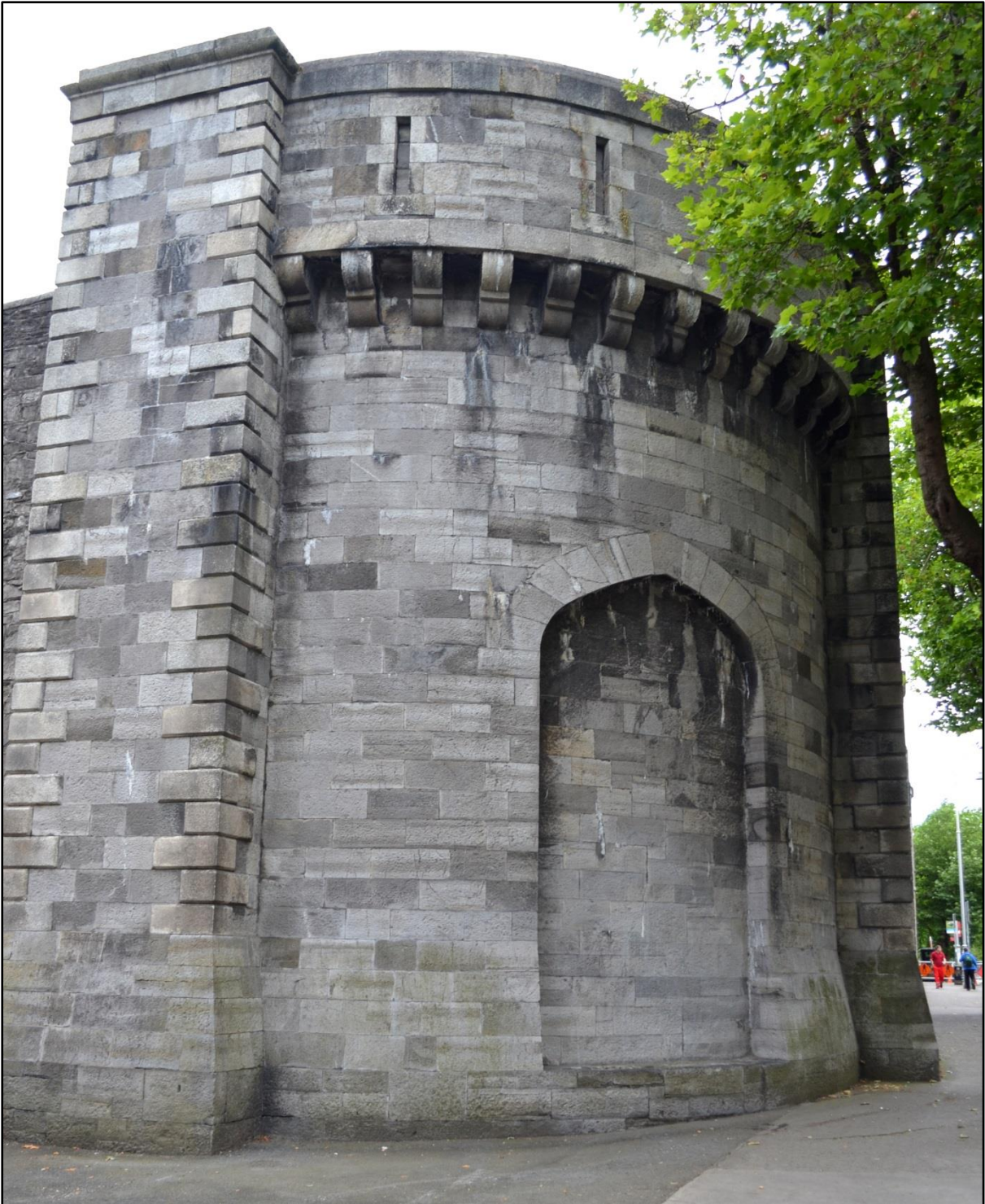
Fig. 48. Kilmainham gaol, Dublin, boundary wall, north-east corner, from the east. While rebuilding half of this gaol in the early 1860s, McCurdy also enlarged the boundary wall and built a pair of matching Norman-Gothic corner towers facing Inchicore road. In an era marked by conformity and standardization in prison design, facades and boundary walls gave architects an opportunity for creativity. Photograph by author, 2014.
