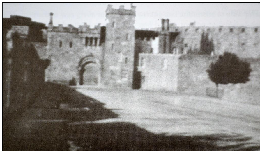
Fig. 51. Kilkenny county and city gaol, entrance gateway, from the east, date unknown but likely during demolition, c. 1948; by this time, the larger central tower had been demolished. William Deane Butler extensively rebuilt Kilkenny's old county gaol between 1850 and 1853; his entrance façade was, like McCurdy's work at Kilmainham, inspired by Norman sources. Photograph by Billy Brett (reproduced in Walsh, 'Hard labour', p. 232). Reproduced with the permission of the journal editor.
