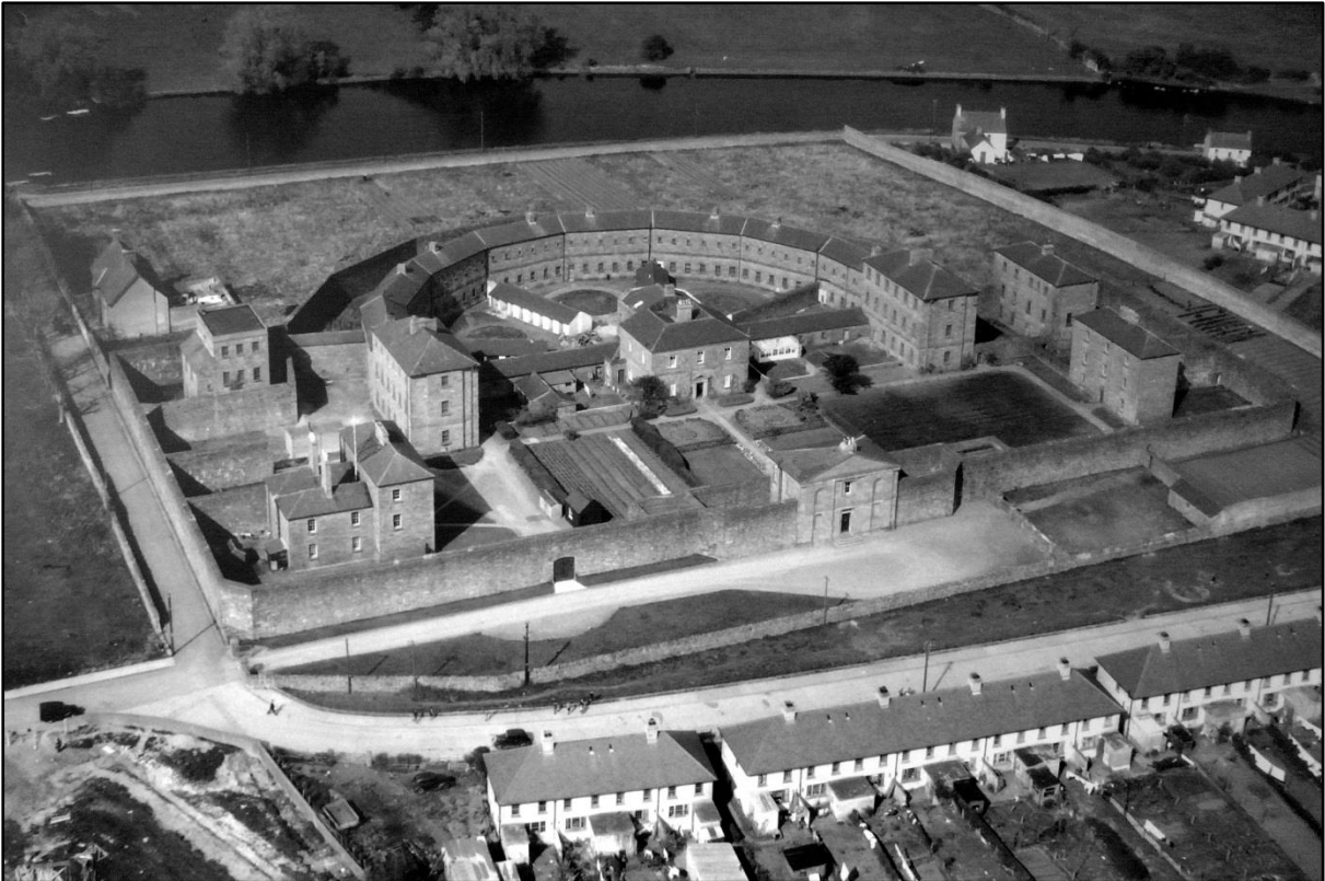
Fig. 34. Sligo gaol, from the south, 1955. While Ingleman's design for Fisherton Anger was rejected on the grounds of cost in 1817, an almost identical scheme was built in Sligo between 1816 and 1818. One of the problems associated with the polygonal plan was ensuring that cells were adequately lighted and ventilated; Sligo gaol was the first in Ireland to solve this problem by having the polygonal range open to the south, bringing sunlight to the entire prison. The approach was originally from the river, but around 1850 a new wide street was built linking it directly with the county courthouse (compare with Fig. 35).
