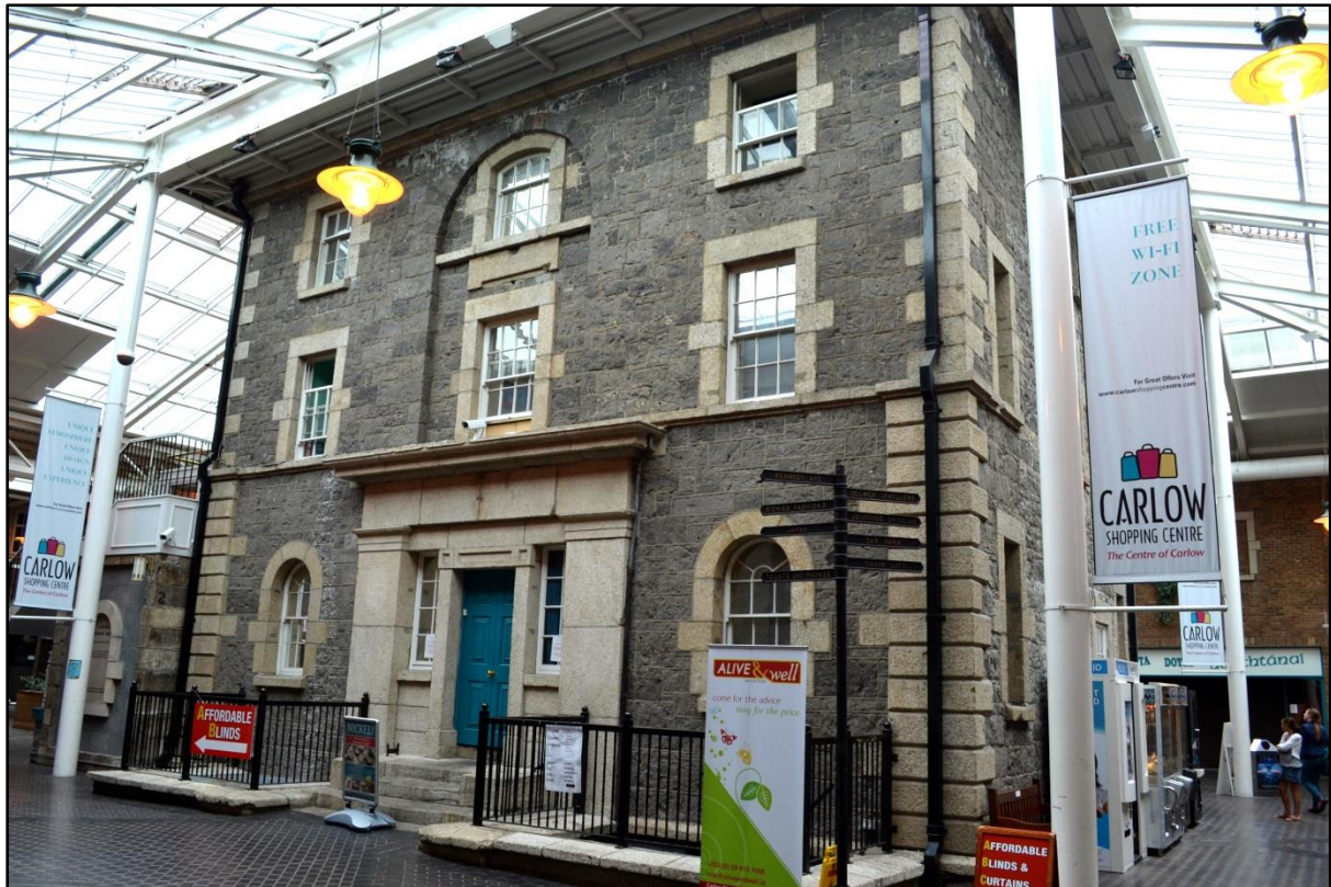
Fig. 40. Carlow gaol, central inspection building, governor's house, and chapel, from the south. Criticism from an assize judge in 1827 pushed the Carlow grand jurors to build a new courthouse (see Chapter 2) and a small radial-plan addition to their gaol. A durable local granite was used for door and window surrounds and for quoins. Photograph by author, 2014.
