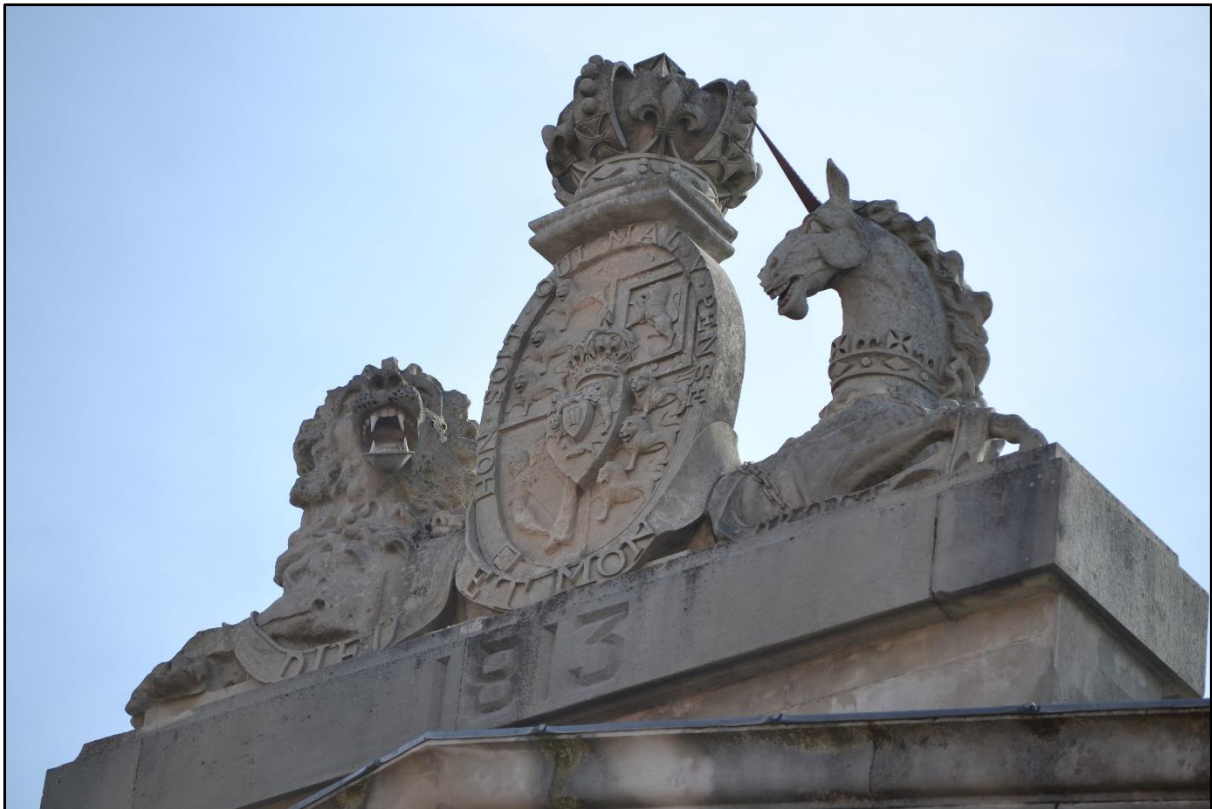
Fig. 46. Derry courthouse, detail showing the coat arms and the date '1813'. C. E. B. Brett notes that the courthouse 'is signed by John Bowden on the back of this coat of arms – a signature visible only from the gutters of the roof' – see Court houses and market houses , p. 90. Photograph by author, 2014.
