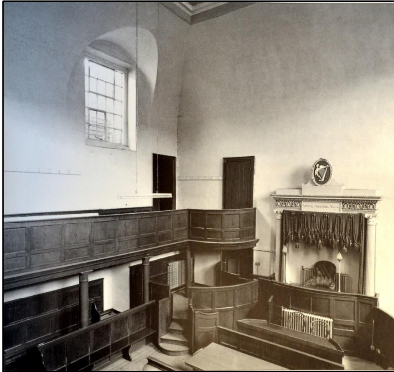
Fig. 29. Courtroom of Clonmel courthouse, c. 1985. As at Philipstown, the courtrooms were double-height and provided galleries for the public and grand juries. Reproduced courtesy of the Irish Architectural Archive.
