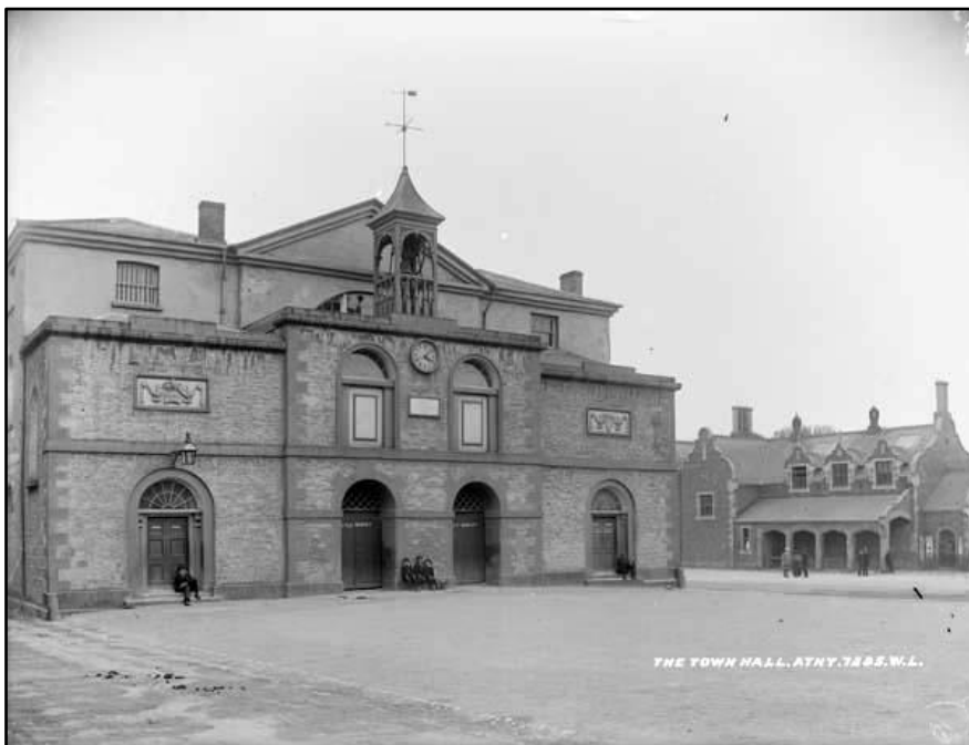
Fig. 30. Athy courthouse and markethouse. This building has a rich and extended history, but it is likely that the relief panels showing the scales of justice date from early nineteenth-century work carried out by Richard Morrison. Much later, an additional storey was built, and the cupola was taken down. To the right, in a Tudor style, is the corn exchange of the 1850s, which later became a courthouse. Reproduced courtesy of the National Library of Ireland.
