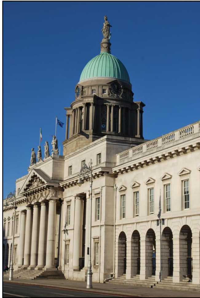
Fig. 18. Custom House, Dublin. The building of this new commercial hub for the city brought a talented architect, James Gandon, to Dublin in the 1780s. Through family connections, it also brought him to Waterford where he designed one of the most influential Irish assize courthouses. Photograph by author, 2011.
